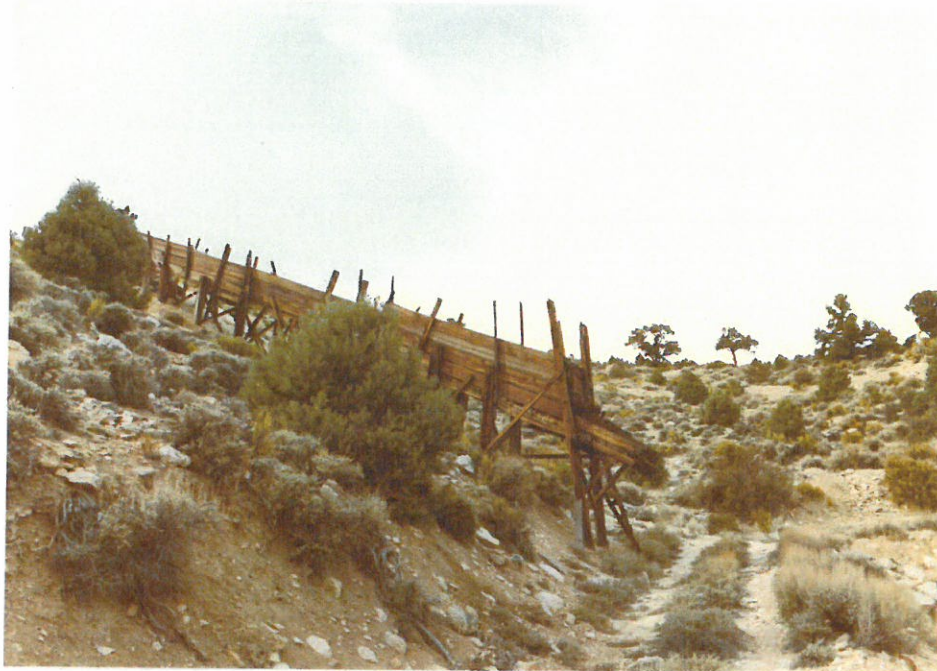
Plate 13. Dumps and small loading chute on the May Day claim (Courbet claim block). An adit at the top of the lowest, lefthand dump (shielded by trees) connects with a shaft which is at the top of the next dump up the hill.
