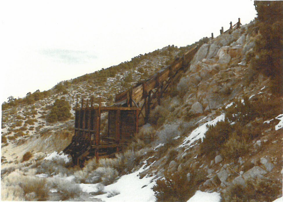
Plate 10. Old ore chute on the Courbet claim, used to load ore from the main adit into carts or trucks for transportation to the mill at Bonnie Claire.
