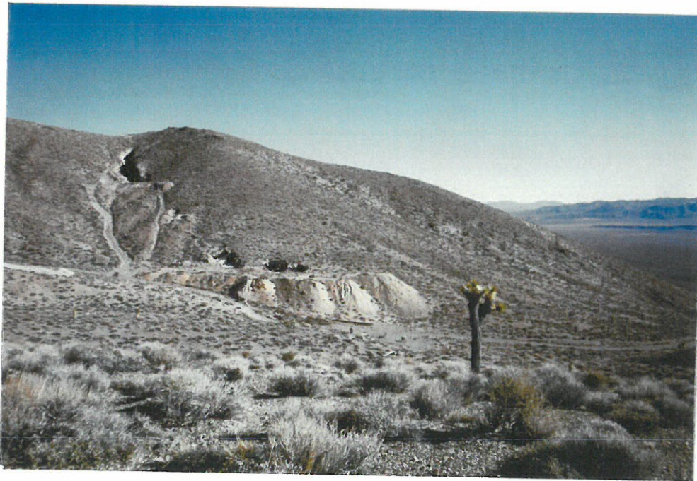
Plate 9. Main dump at the Rattlesnake mine. The workings follow the trend of the vein along the surface.
