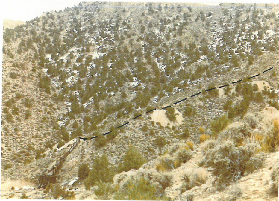
Plate 11. Courbet claim showing three dumps and the ore chute. The dashed line shows the trend of the vein along the surface. Adits cut into the vein from the lower dump and from the main dump which is mostly behind the ridge in this photograph.
