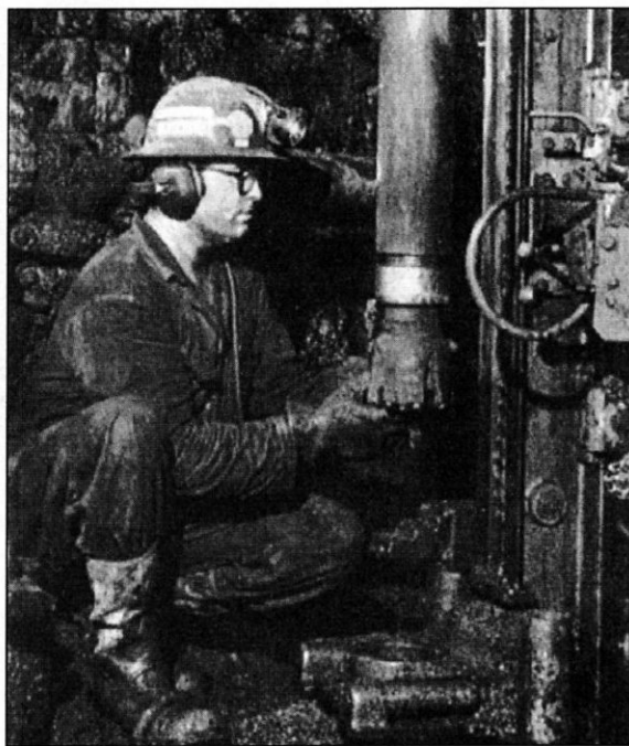
FIGURE 1.15 ITH drilling, 165 mm blast holes, INCO, Canada
